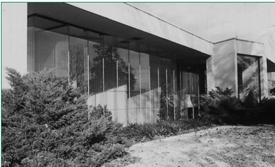
Headquarters of precast concrete producer Trenwa, Inc., Fort Mitchell, Ky., features "Cool Community" concepts such as southwestern-exposed massive concrete wall near glass exterior wall and white aggregate reflecting yard. Photo courtesy of Concrete Products magazine.
