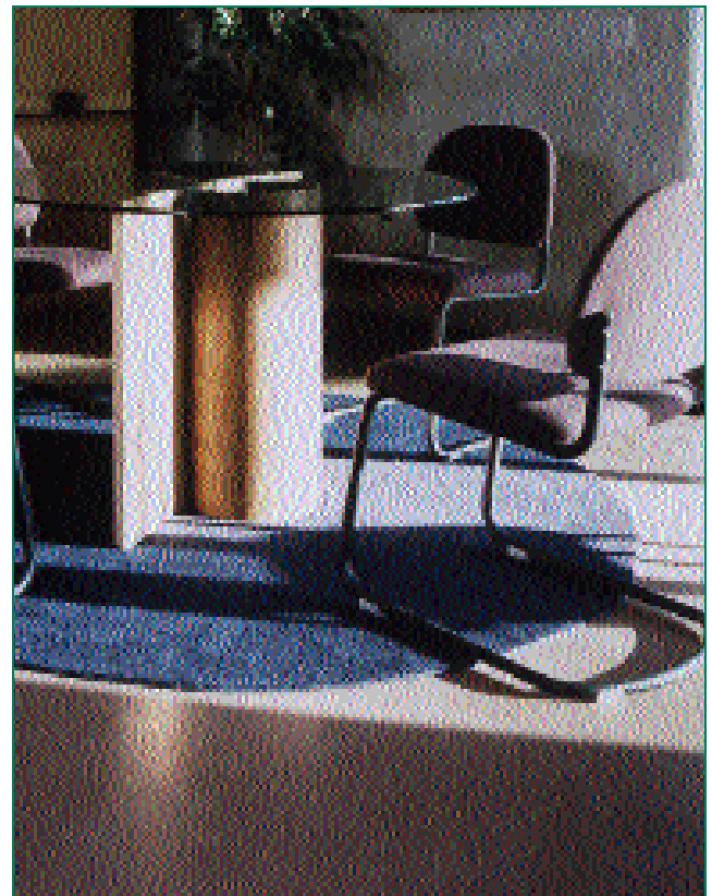
Attractive cast-in-place flooring can be colored and textured in a variety of ways.
